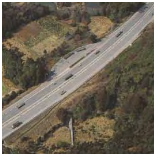
Photo 1 Application for road construction
